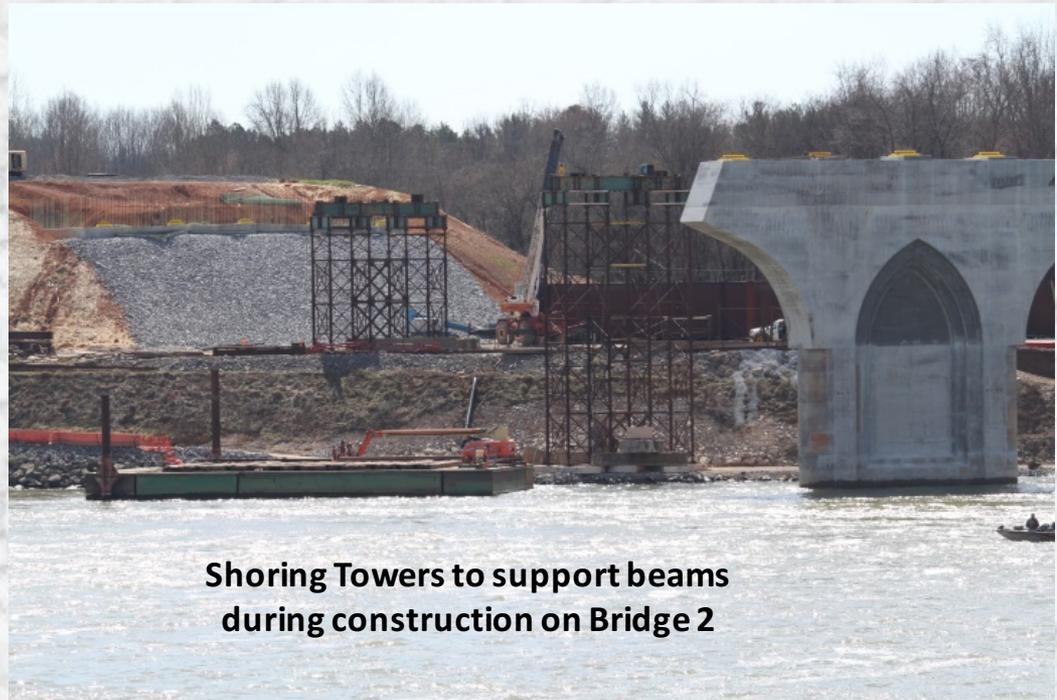
**Shoring Towers to support beams during construction on Bridge 2**
